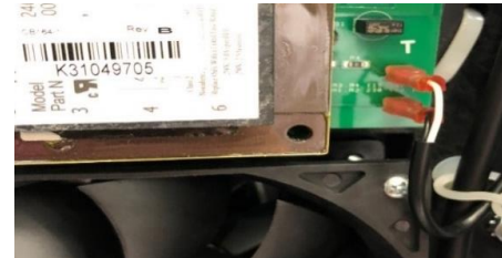
Figure 15.B. Installed Terminals to Fan Board
