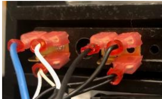
Figure 17.6. Intensity 10 230V Terminal Wires
