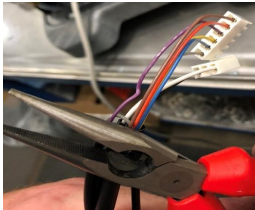
Figure 12. Separated Wire Harnesses
