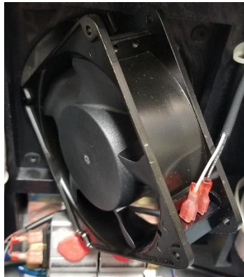
Figure 15.A. Installed Terminals to Fan
